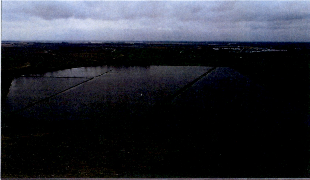
Photo 1. Helena WWTP Aerial view of all cells
