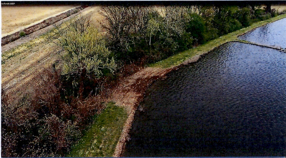
Photo 5. Helena WWTP Cell 3 South-west corner aerial view
