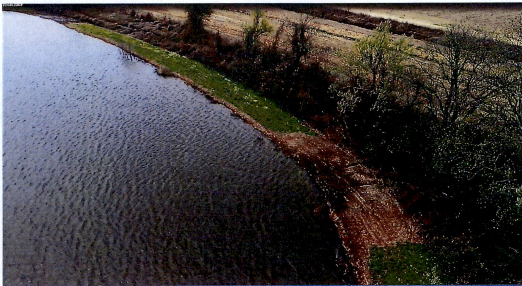
Photo 6. Helena WWTP Cell 3 SW corner frontal aerial view
