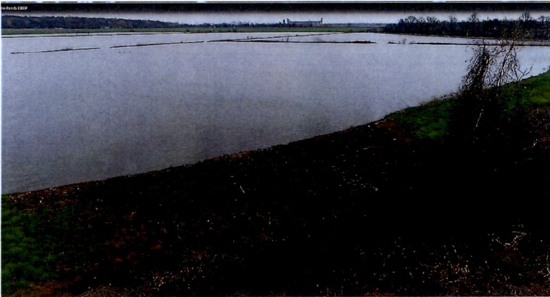
Photo 4. Helena WWTP Cell 3 South Wall Anterior View
